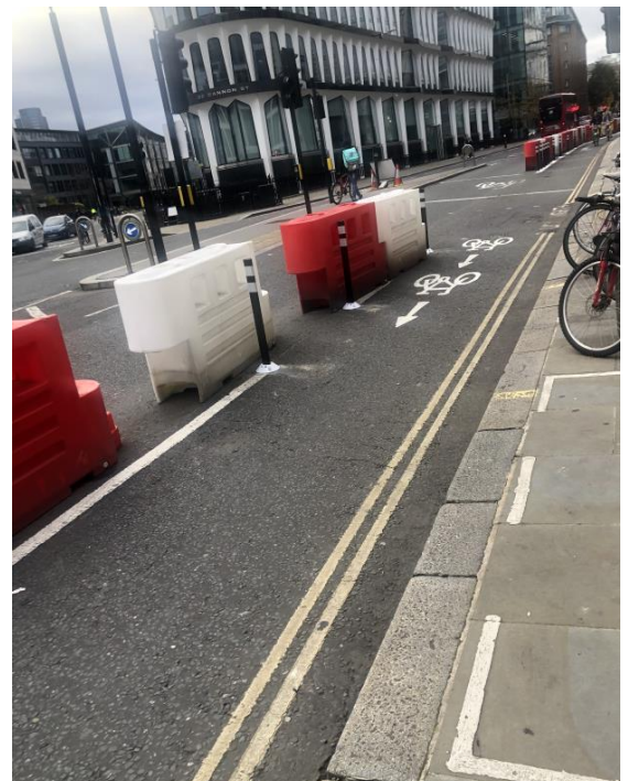
FIGURE 11 EMERGENCY CYCLE LANE, CANNON STREET, CITY OF LONDON. IDENTIFYING ROAD BLOCKS USED FOR SEGREGATION
