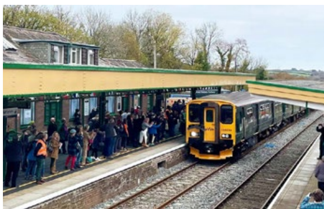
Okehampton station on the first day of the restored Dartmoor Line, November 2021
